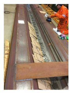
Fig. 7: Installation of the sensors on a sheetpile. The sensing elements are covered with an individual protective cover which does not interfere with their function as strain sensors.
